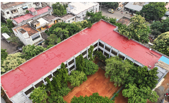
Before cool roof
