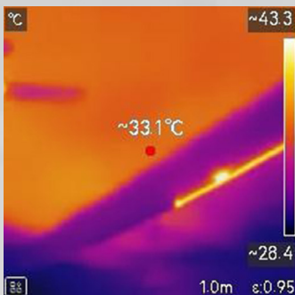
Before – Ceiling Surface Temperature
