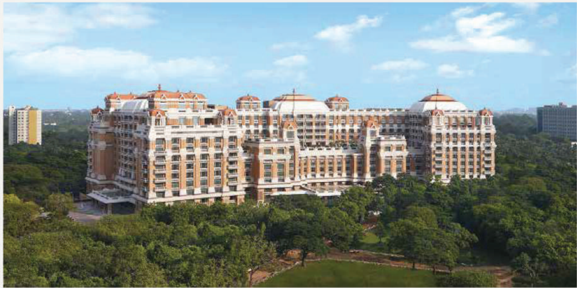
Figure 53: Overview of green building actions by ITC Grand Chola in Chennai (GRIHA, 2018)
